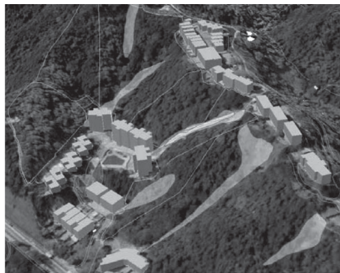
Figure 6. Residential buildings affected by landslide hazards at Sha Tin Heights (after Wong & Ho 2005).
