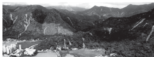
Figure 11. Natural terrain landslides at Tung Chung, Lantau Island during the June 2008 rainstorm.
